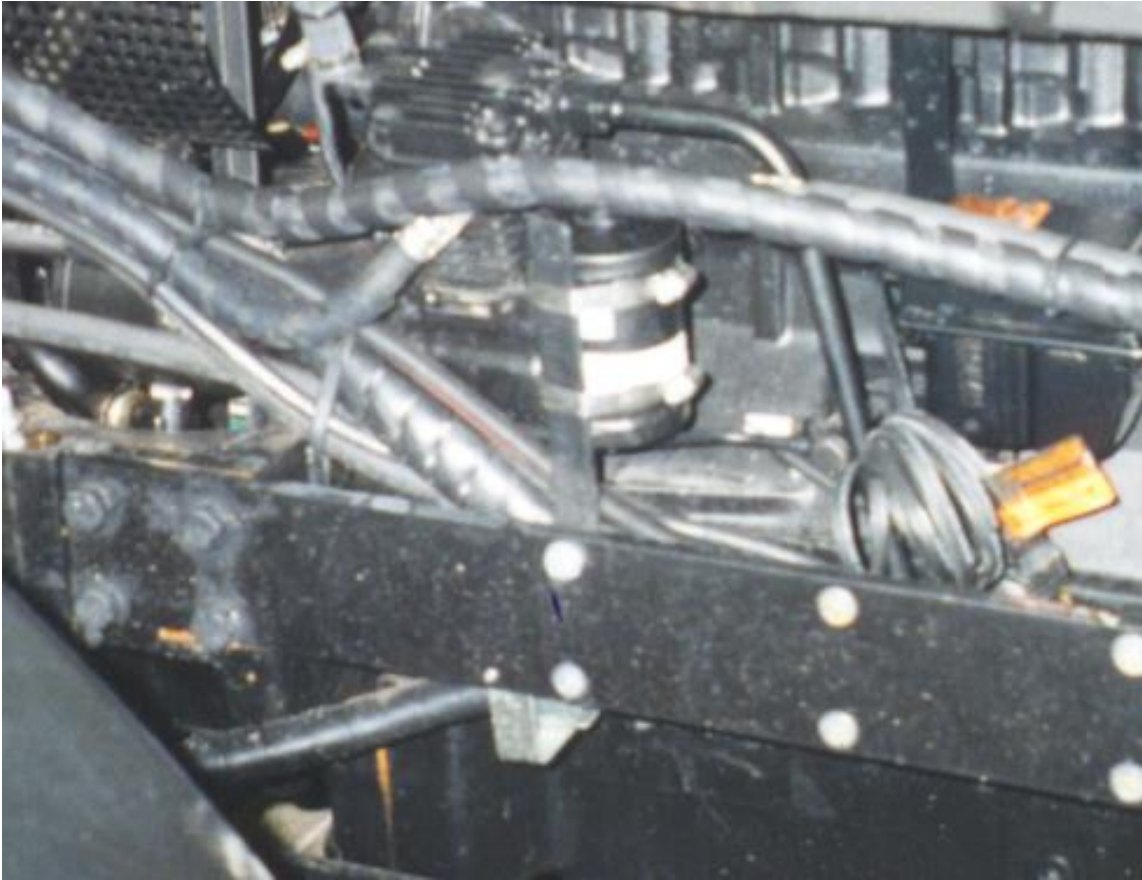
Drier and bracket in place showing hoses.
